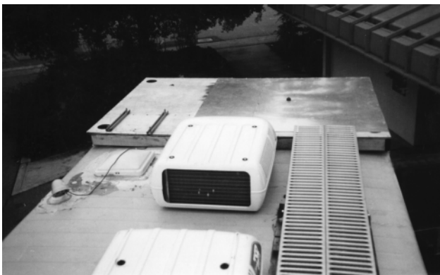
Figure 3. Antenna mounting plane and catwalk.
